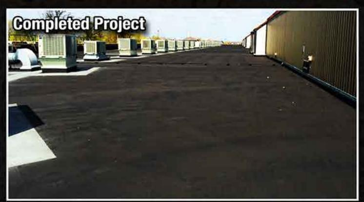
Liquid Rubber Professional was specified on this project, due to its high performance, seamless finish and rapid spray application rate. Refurbishment works to the existing failing single—ply roof consisted of the area being cleaned, then detailed using Liquid Rubber Professional Brush & Roller, embedded with Liquid Rubber GeoTextile to give further reinforcement.
