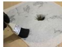
Brush Joint Tape into Primer to embed
