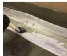
Brush Joint Tape into Primer to embed
