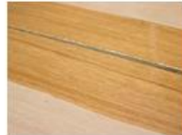
Primer poured onto and into joint to re-bond
