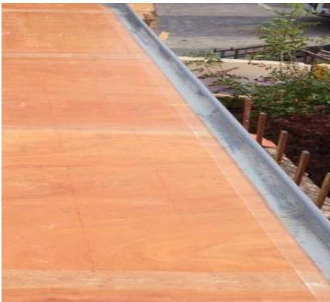
New GRP trim installed and reinforced using EcoProof Detailing Primer and EcoProof Joint Tape.
