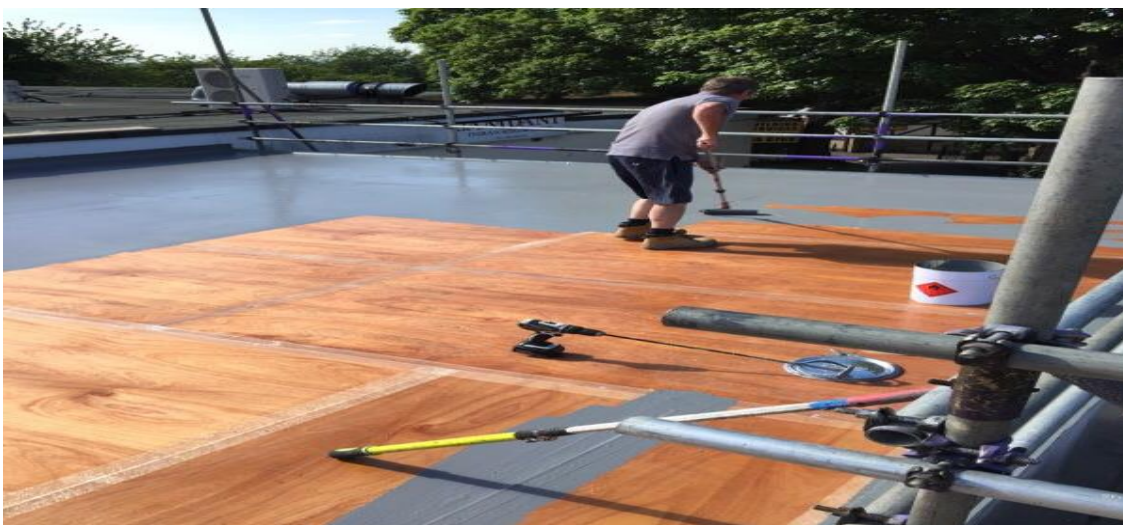
Above: First coat being applied at 1kg per m 2 .
