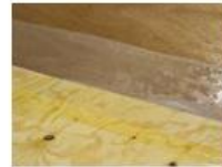
Brush Joint Tape into Primer to embed
