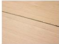
De-bonding joint cleaned out
