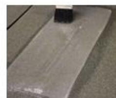
Joint Tape embedded into Primer
