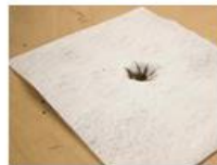
Primer poured onto and into joint to re-bond
