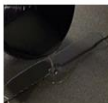
Primer poured onto and into joint to re-bond
