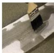
Brush Joint Tape into Primer to embed
