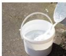
Catalysed product poured into aggregate
