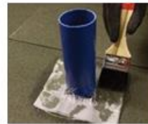
Joint Tape brushed into primer
