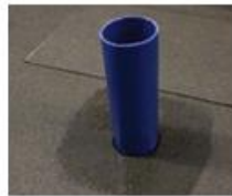
Primer applied to surface and pipe
