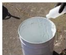
Catalyst added to base product and mixed
