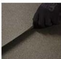
De-bonding joint cleaned out
