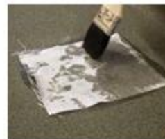
Joint Tape embedded into Primer
