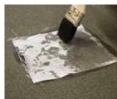
Joint Tape embedded into Primer
