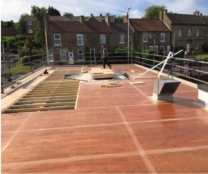
Picture shows new deck being laid.
