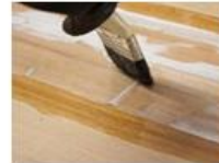
Brush Joint Tape into Primer to embed
