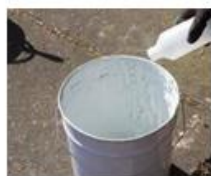
Catalyst added to base product and mixed
