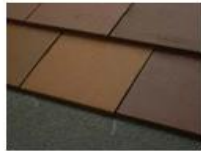
De-bonding joint cleaned out
