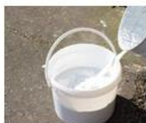
Catalysed product poured into aggregate
